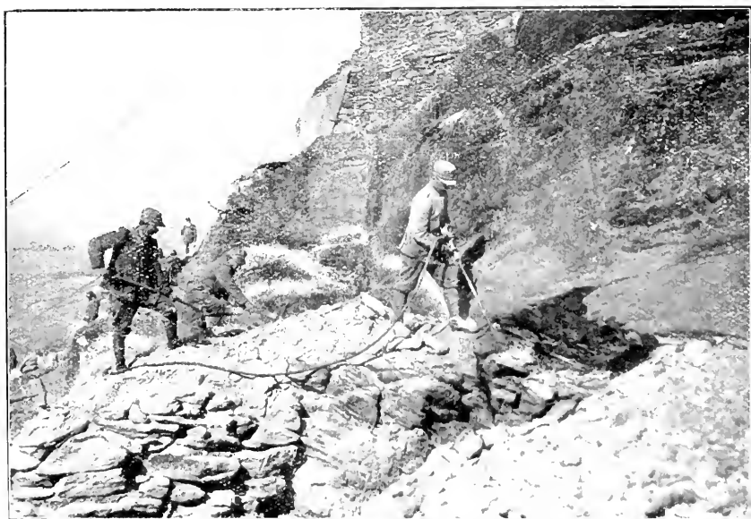
ROCK-PERFORATING MACHINE ON HILL 1050.
